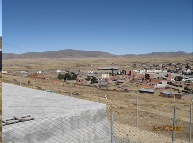
Water tank, town of Batallas
