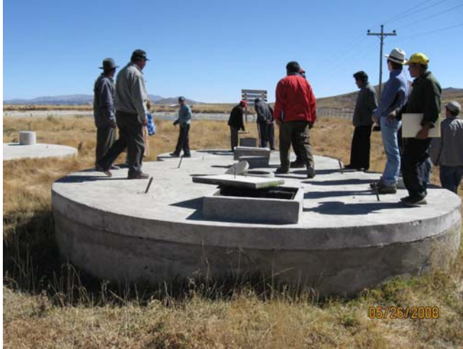
Batallas Wastewater Treatment Plant
