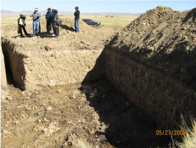
Excavation for tank, distribution line
