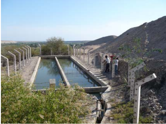
Intake for Inclan water system with high arsenic levels
