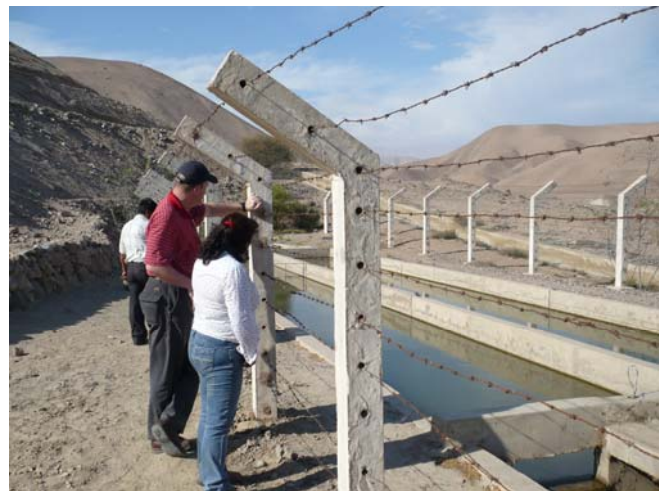
Water system inlet for community of Inclan in the Sama Valley
