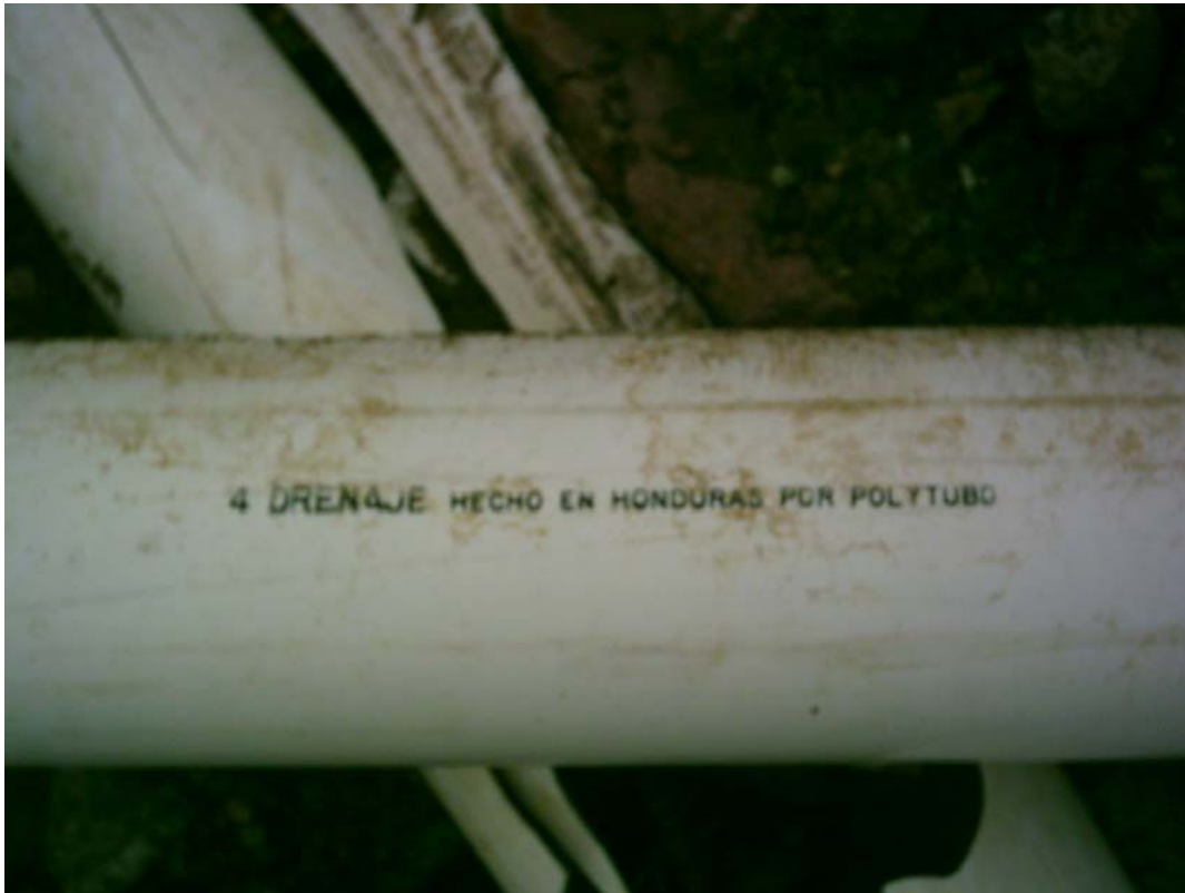
As can be noted, the old main transmission line was drainage pipe (DR 64)
