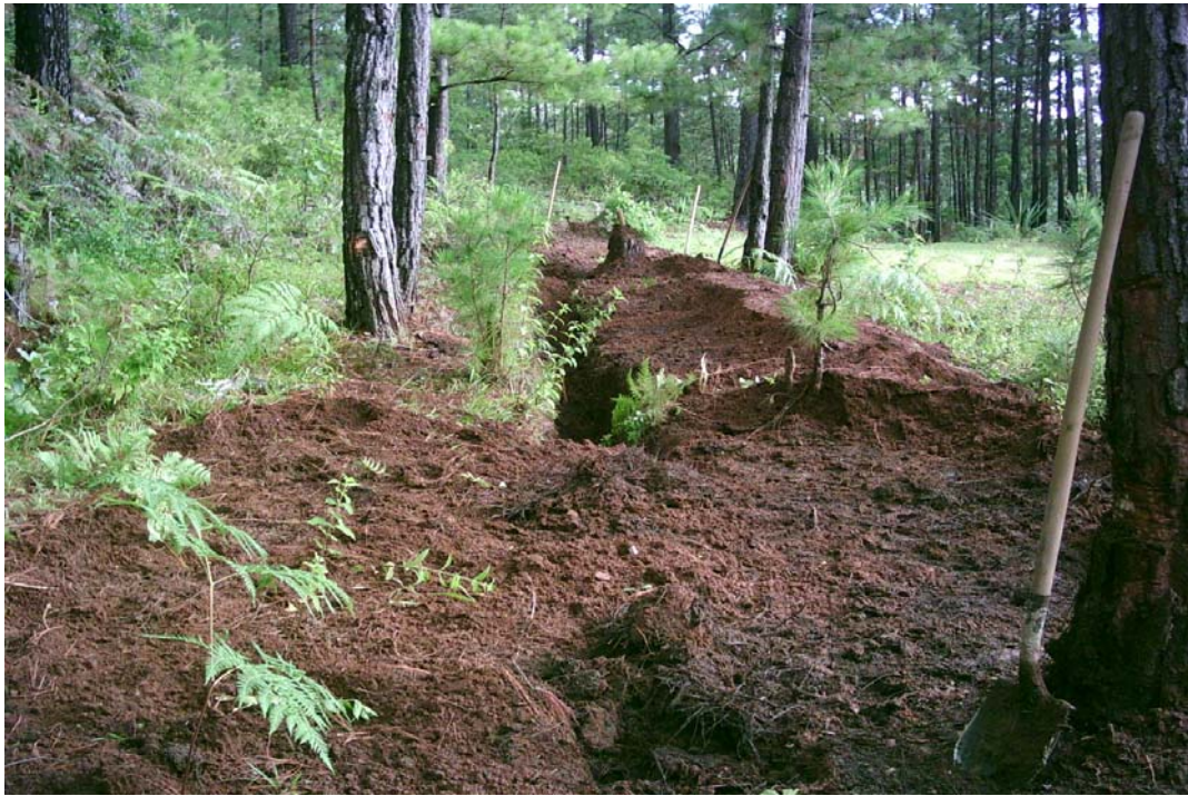
Once laid, the pipe trench is backfilled
