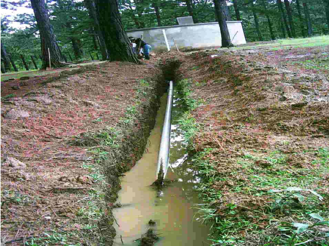
The waterline arriving at the water tank
