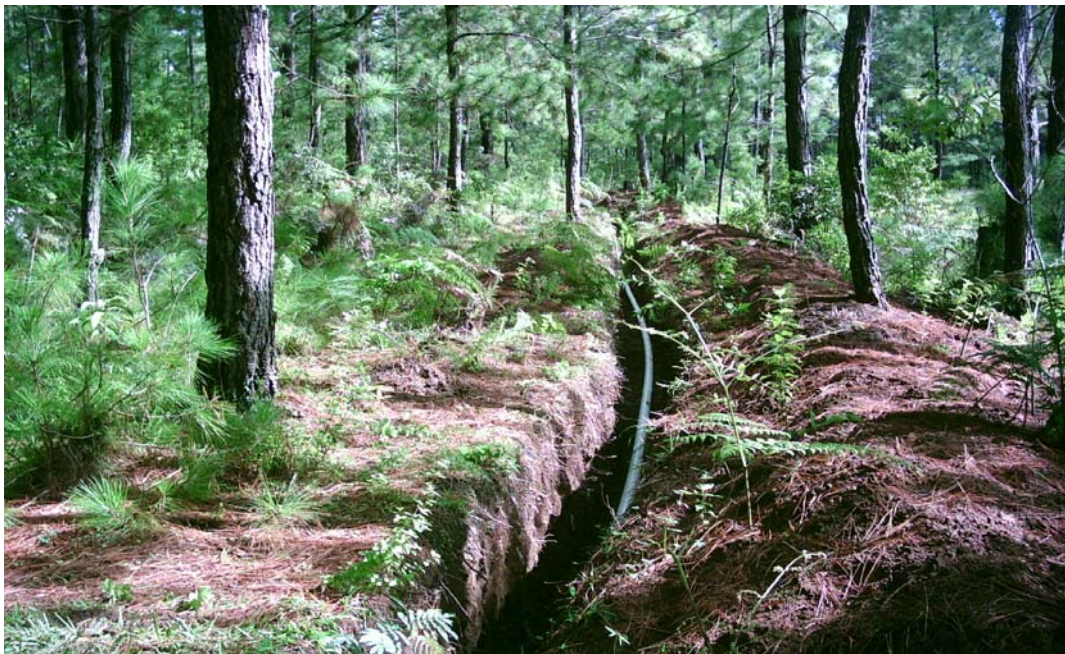
Section of the mainline between spring source and storage tank
