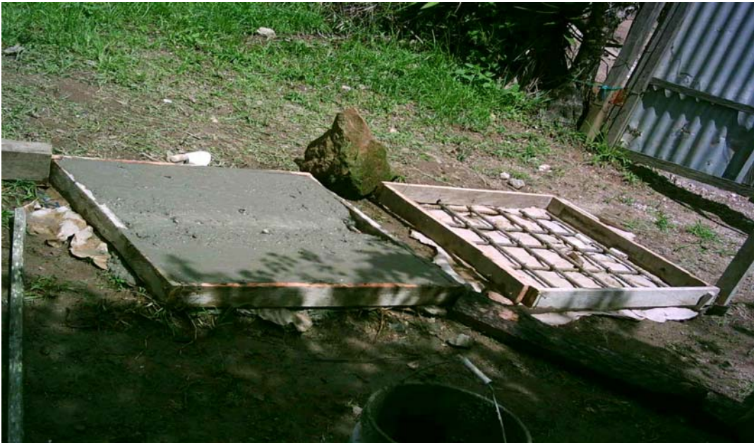
Construction of the covers to the valve boxes
