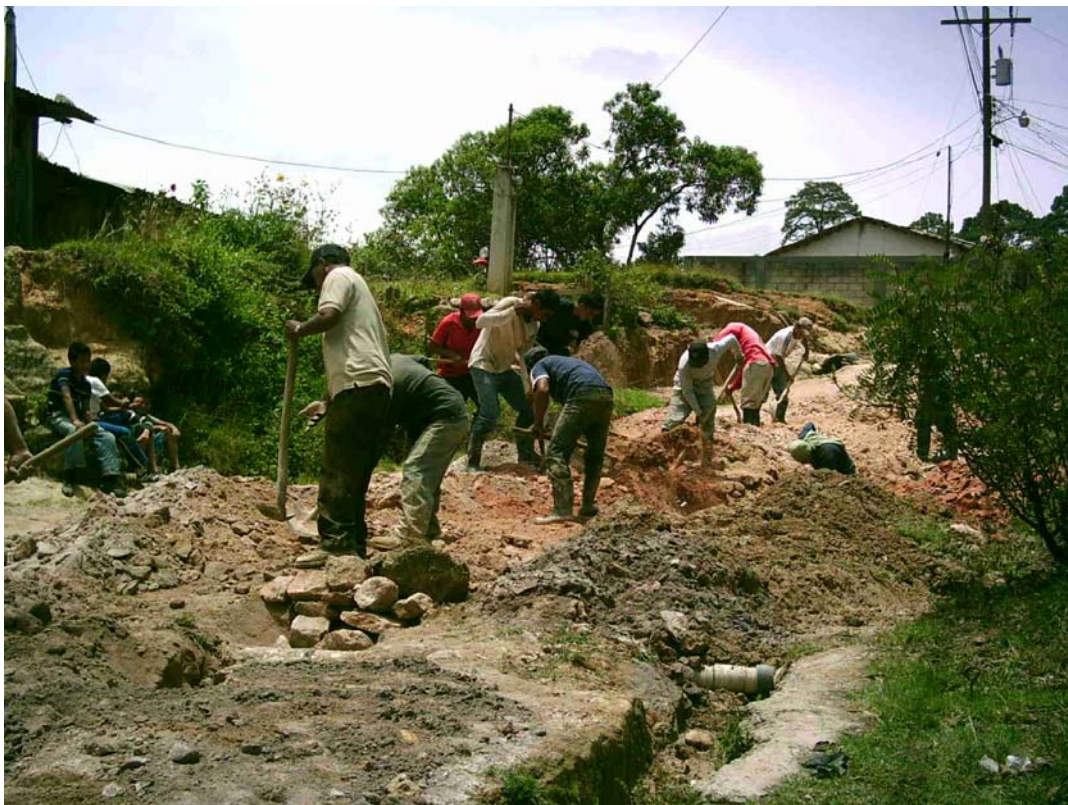
Backfilling of pipeline by community members
