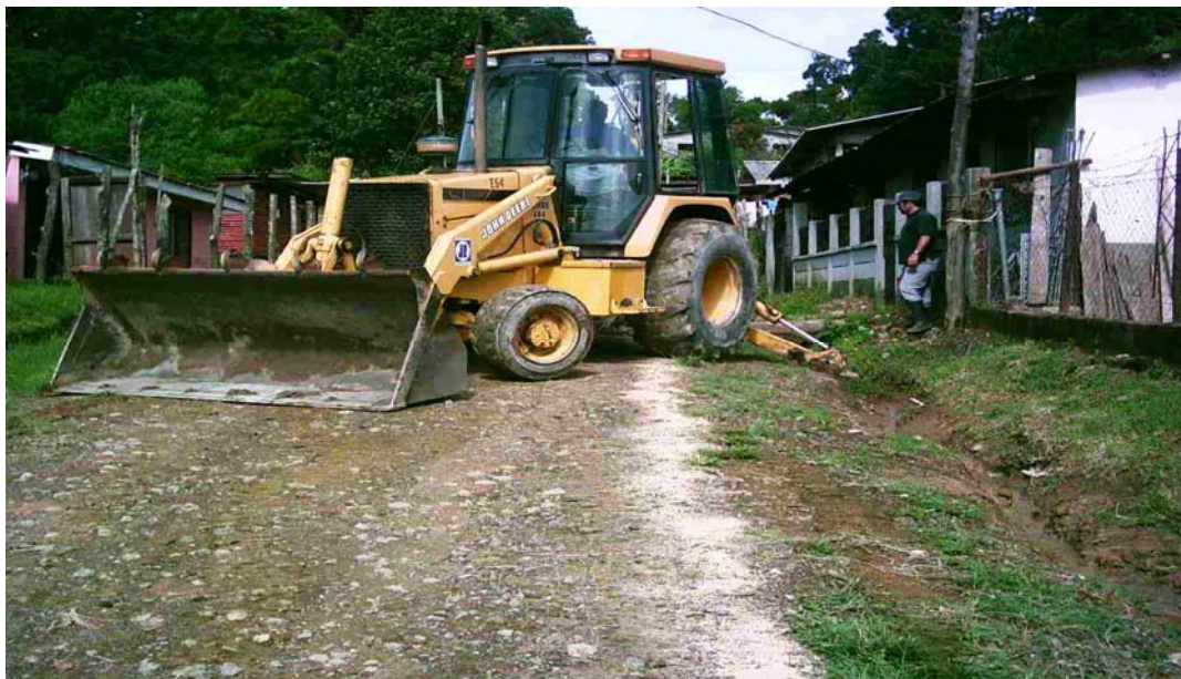
This 4" PVC SDR26 pipe was located in an extension of the distribution system to provide water to another sector of the community. Due to very hard soil conditions it was necessary to use a backhoe in this area.
