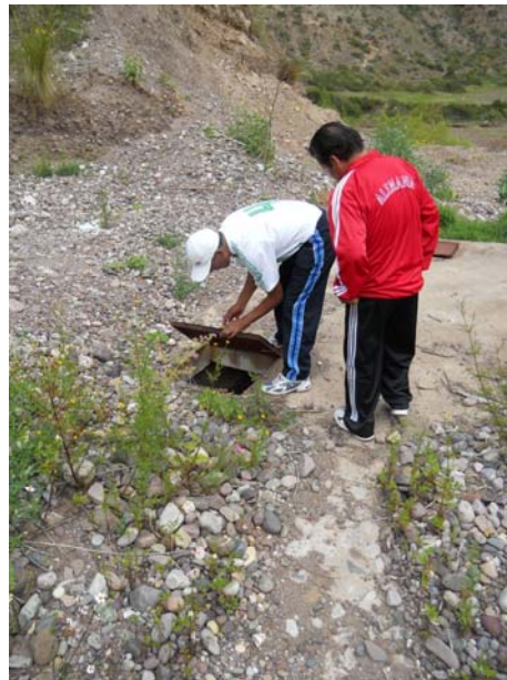
Guillermo and Zacharias inspecting septic tank at lower site
