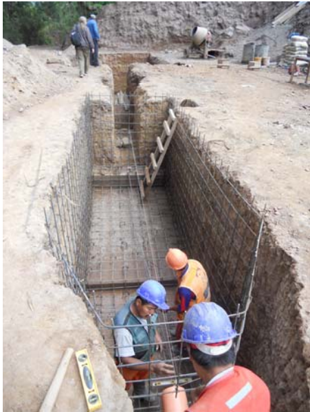
Pumahuanca wastewater treatment system under construction
