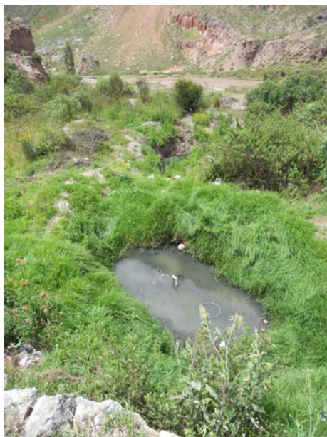
Site of failed septic system where new percolation pits will be constructed
