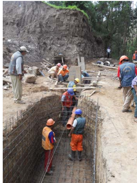
Pumahuanca wastewater treatment system under construction
