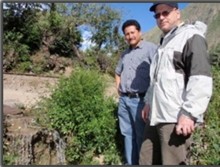
Discharge from one of Ollantaytambo outfalls
