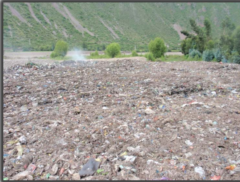
Calca Upper WWTP Site
