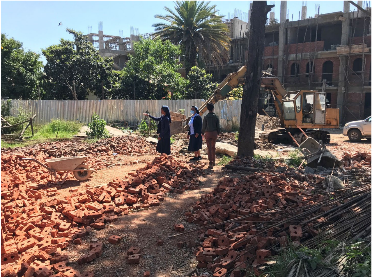
Fig. 20 – Construction at St. Catherine's
