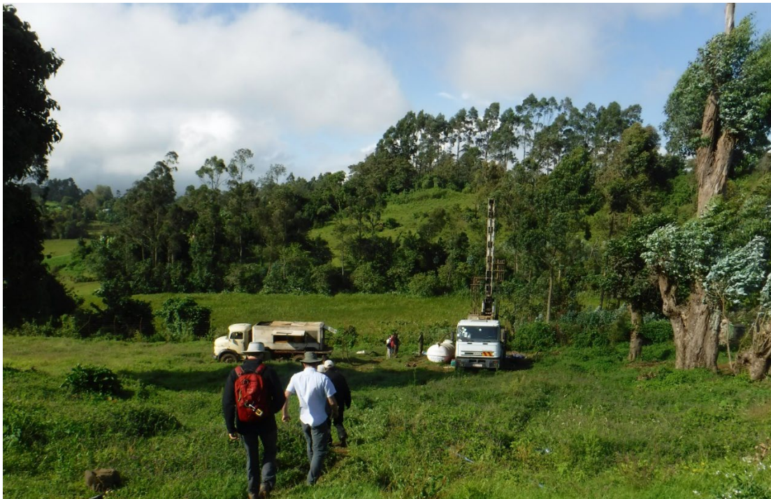
Fig. 6 – AEID drilling for water at the Maji District Hospital
