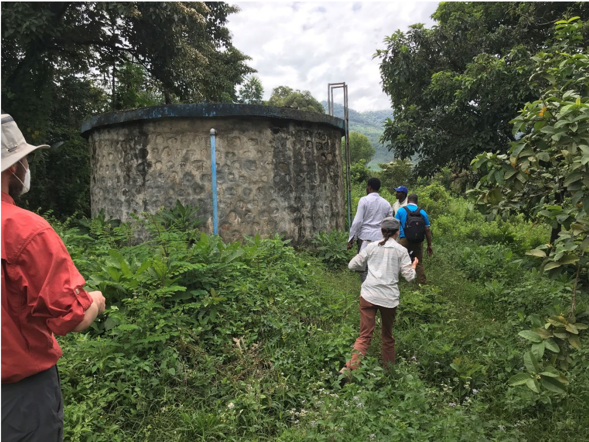
Fig. 7 – The Tum water storage tank that supplies the HCF
