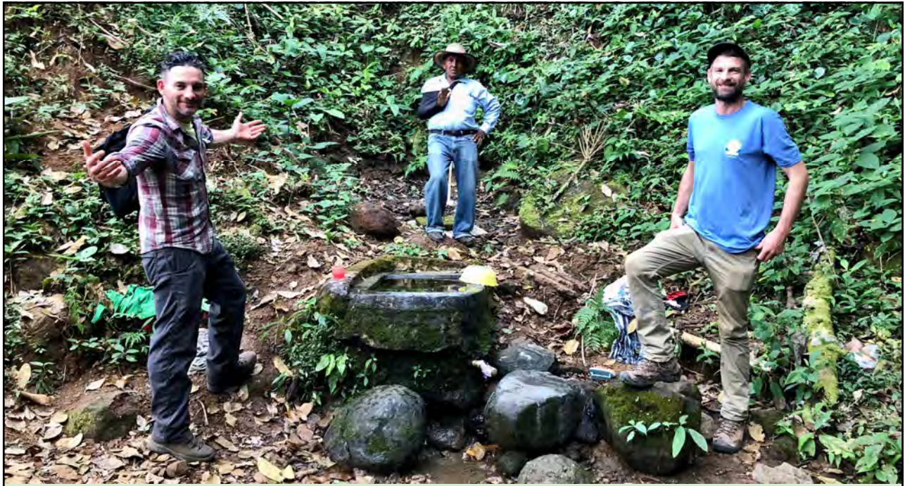
Zapote: WEFTA team visiting the spring capture site Nicholas built. It is still functioning well.
