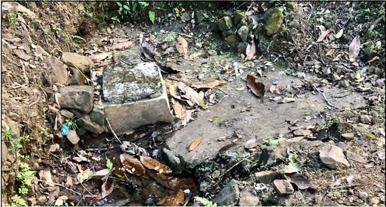
Alto Estrella: the community constructed low-profile spring capture
