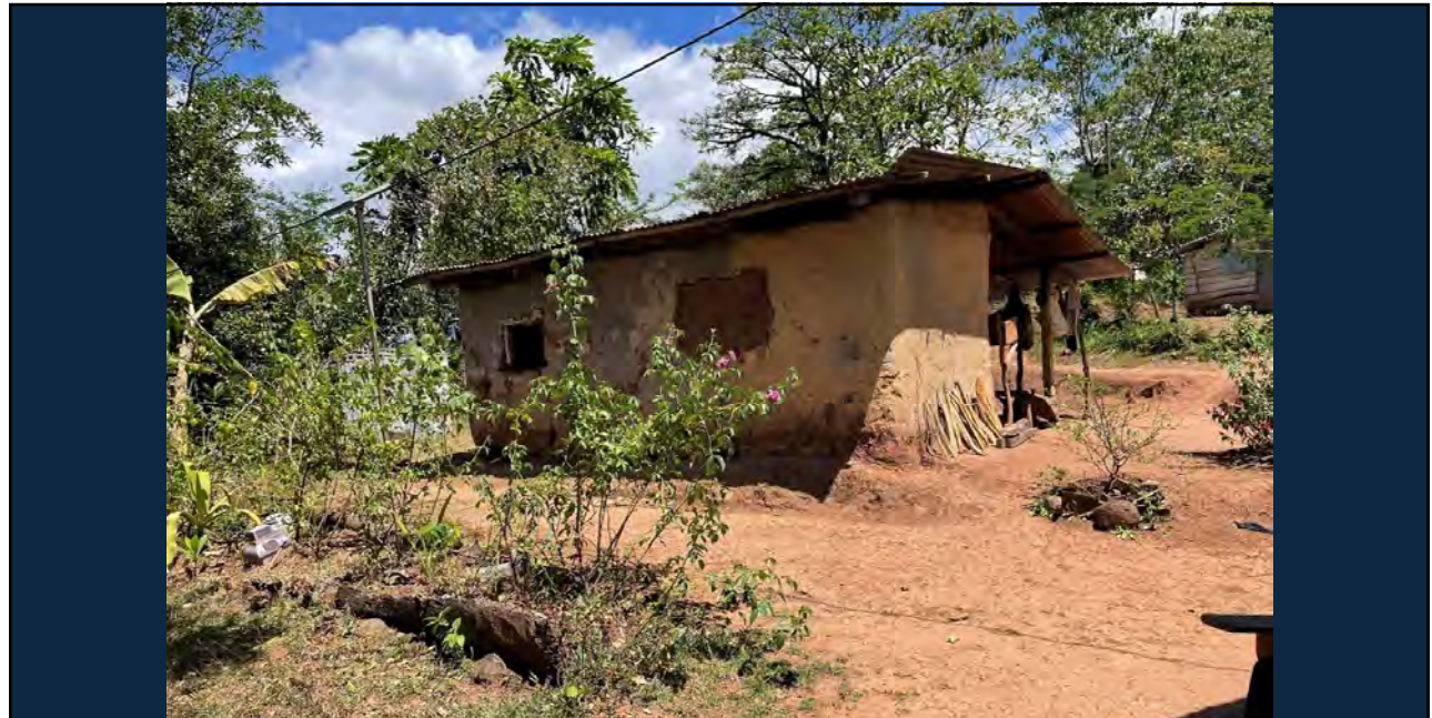
A typical adobe or “quinche” house. Quinche, which is mud and dried grass, was the construction material before communities were able to receive concrete and blocks to build their homes.
