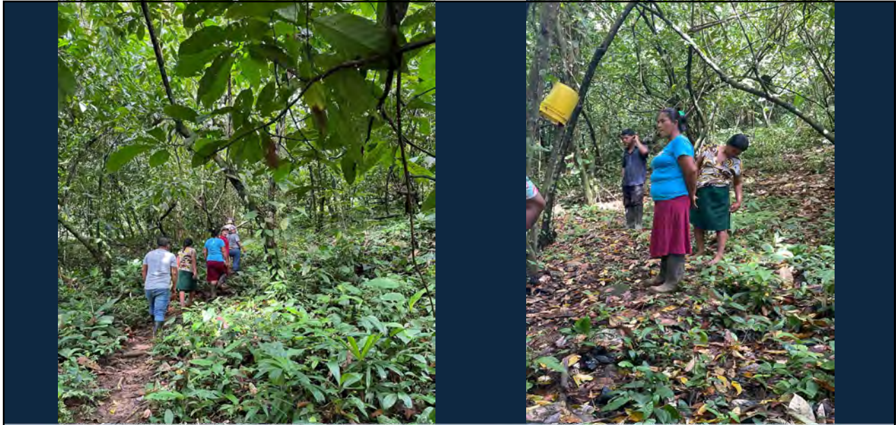
Many community members who were part of the work crew that mixed the cement to build the system made the trek to the spring as well. Since most of the men work outside the community because many women were part of the actual construction of the water system.
